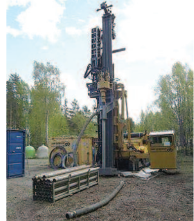
Figure 10: Borehole drilling in Sweden (source: SKB/Alf Sevastik Kustbild)
