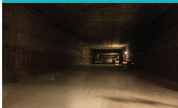
Figure 6: Underground facilities at the WIPP plant in New Mexico (source: WIPP)
